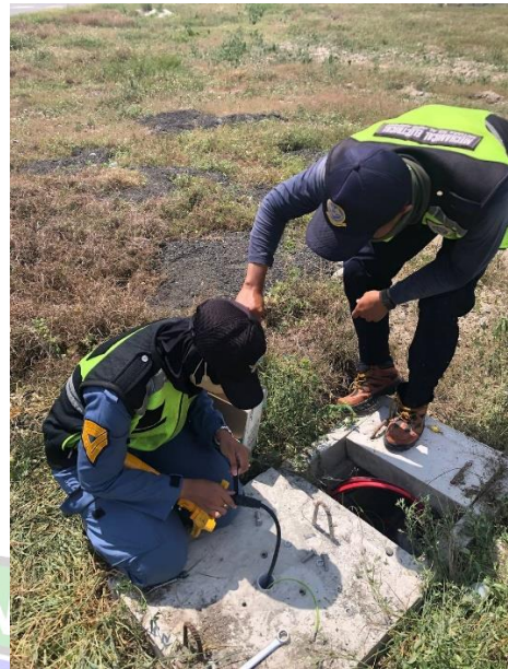
Pemasangan lampu taxiway led baru
