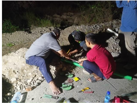
Gambar 4. 25 Proses Crimping
