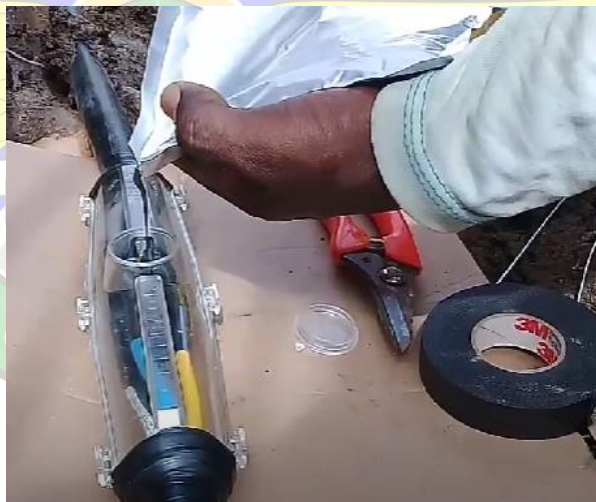
Gambar 4. 24 Proses pemberian resin
