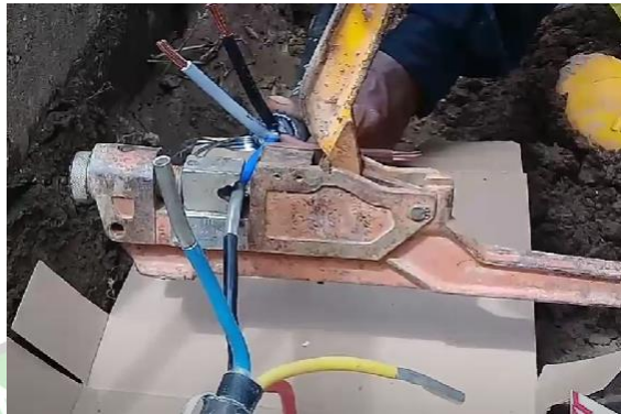
Gambar 4. 21 Proses Crimping
