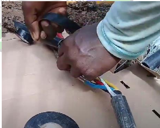
Gambar 4. 22 Proses rubber kabel
