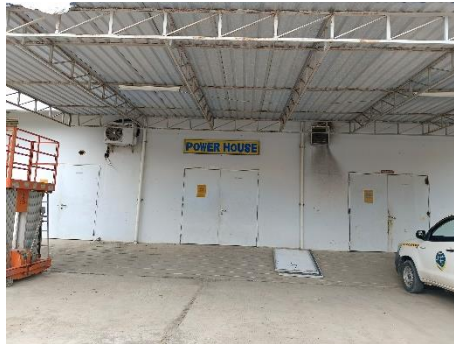
Gambar 4. 6 Gedung Power House Bandara Kalimantan
