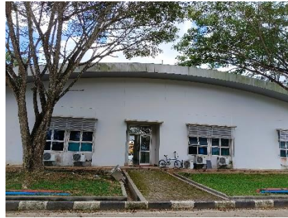
Gambar 4. 8 Gedung Maintenance Bandara Kalimarau
