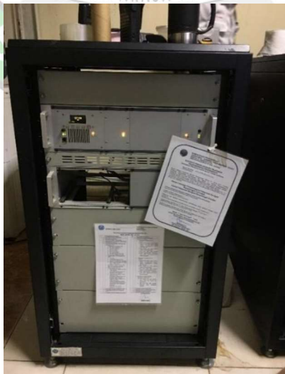
Gambar 3. 7 Transmitter ATIS Kendari
