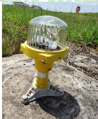
Gambar 2. 18 Runway Edge Light Elevated Sumber : Bandara Internasional Juwata Tarakan
