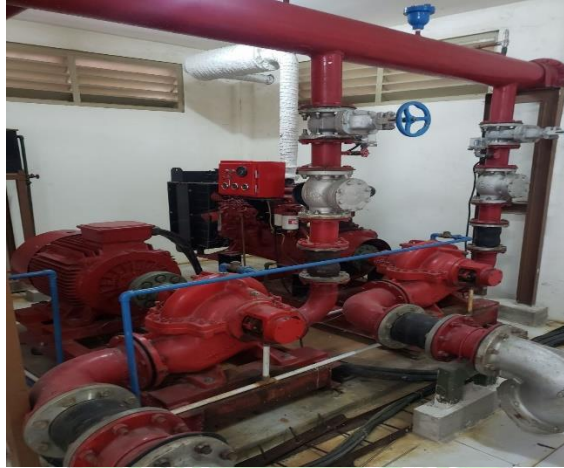
Gambar 2. 32 Pompa Hydrant
