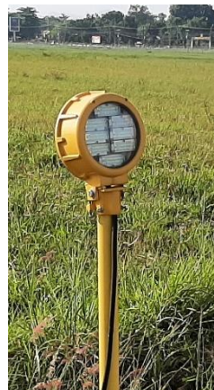
Gambar 2. 3 Sequence Flashing Light (SQFL)
