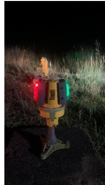
Gambar 2. 6 Threshold Light dan Runway End Light Elevated
