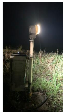
Gambar 2. 4 Runway Threshold Identification Lights
