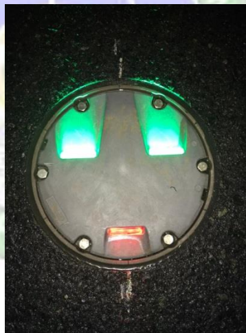
Gambar 2. 5 Threshold Light dan Runway End Light Insert
