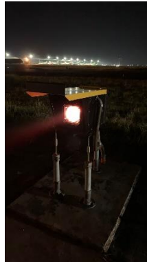
Gambar 2. 9 Precision Approach Path Indicator (PAPI)
