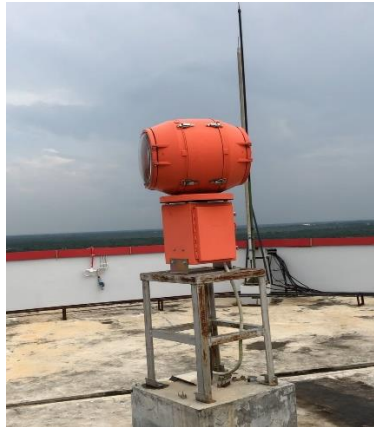
Gambar 2. 17 Rotating Beacon
