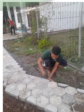
Gambar 4.18 Meratakan conblock
