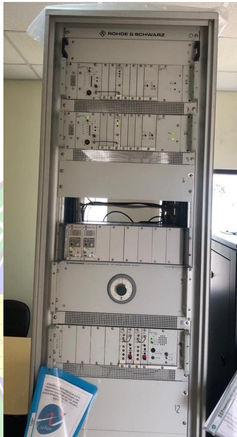
Gambar 3.2 VHF A/G Secondary ADC
