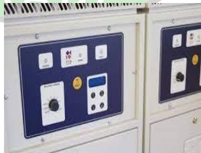
Gambar 2. 17 Constant Current Regulator
