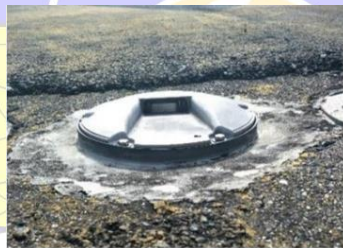
Gambar 2. 7 Threshold Light / End Light
