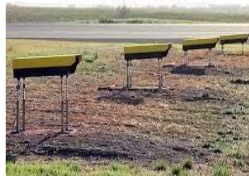
Gambar 2. 8 Precision Approach Path Indicator (PAPI)
