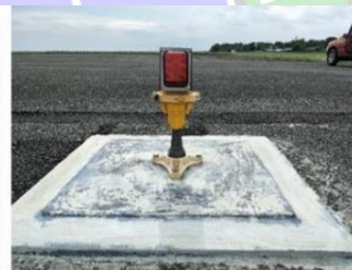
Gambar 2. 7 Threshold Light / End Light
