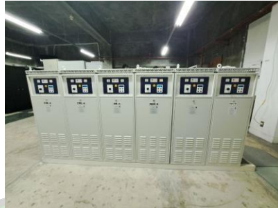
Gambar 3. 3 Constant Current Regulator
