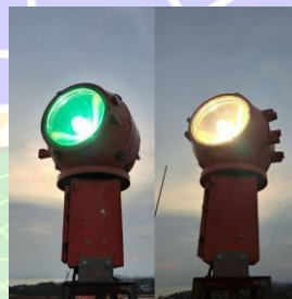
Gambar 2. 16 Rotating Beacon
