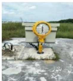
Gambar 2. 13 Runway Threshold Indicator Light
