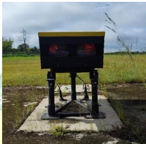
Gambar 2. 14 PAPI ( Precision Approach Path Indicator ) Sumber: Bandara Udara H. Asan Sampit
