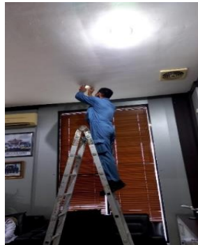
Penggantian Lampu Downlight
