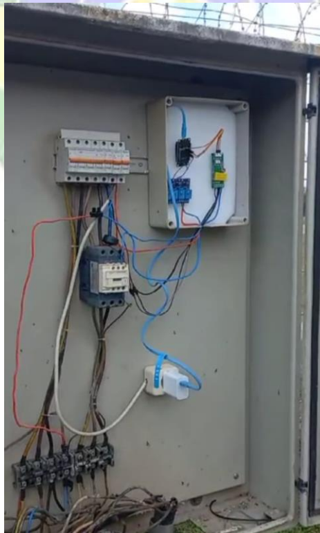
Gambar 4. 4 Panel sesudah dipasang Alat
