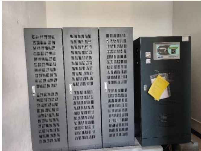
Gambar 2. 9 Uninterruptible Power Supply Sumber: Bandar Udara H. Asan Sampit
