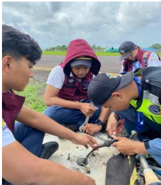
Penggantian Trafo Lampu Taxiway
