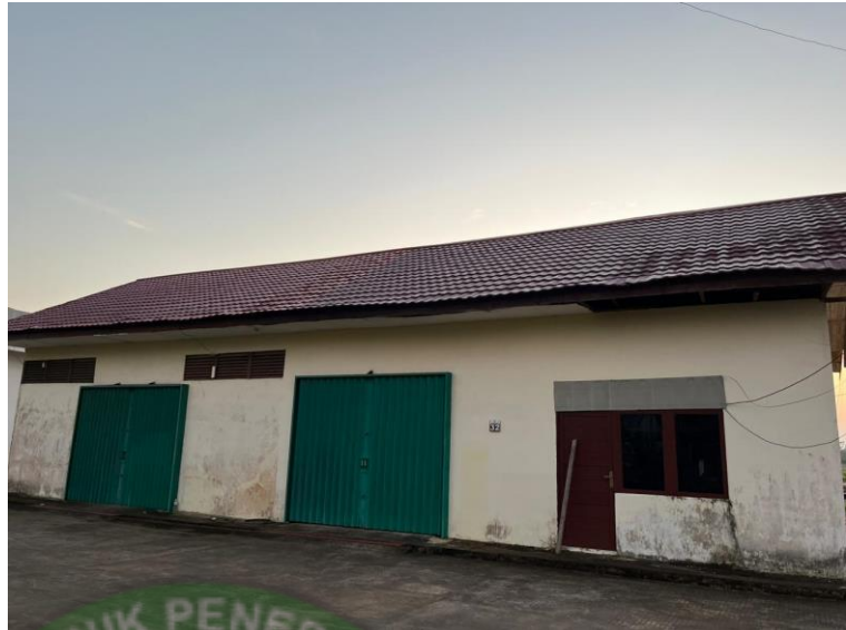
Gambar 4. 10 Gedung Power House
