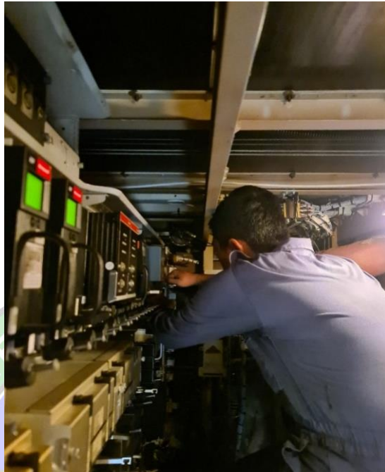
Gambar 4.14 Replace XCVR-HF1
