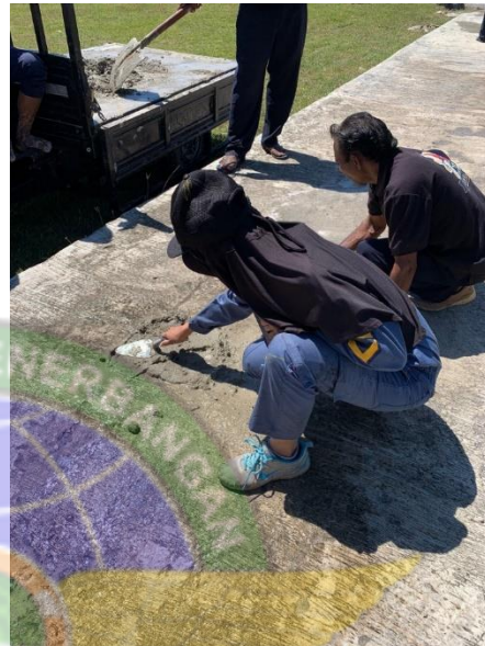
Gambar 4.22 Proses Patching
