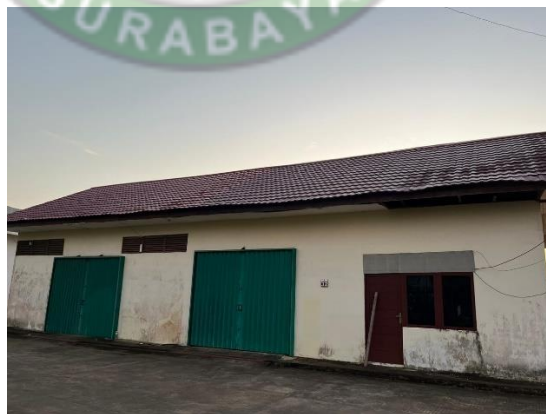
Gambar 4. 6 Gedung Main Power House
