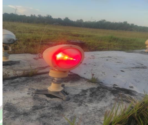
Gambar 2. 12 Runway End Light Elevated
