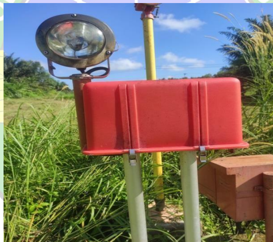
Gambar 2. 19 Sequence Flashing Light
