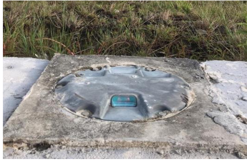
Gambar 2. 11 Runway End Light Insert
