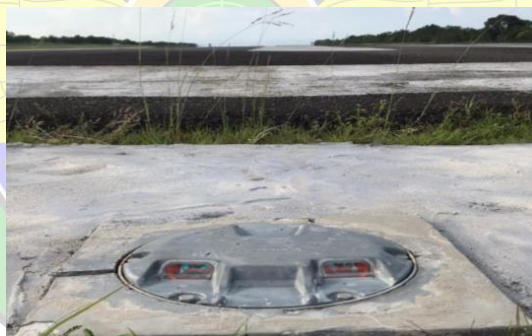
Gambar 2. 8 Lampu Threshold Insert
