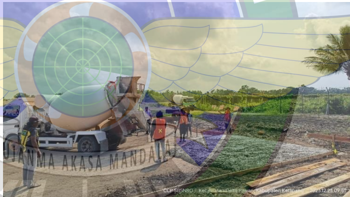
Gambar 4.33 Proses Pengecoran Ready Mix
