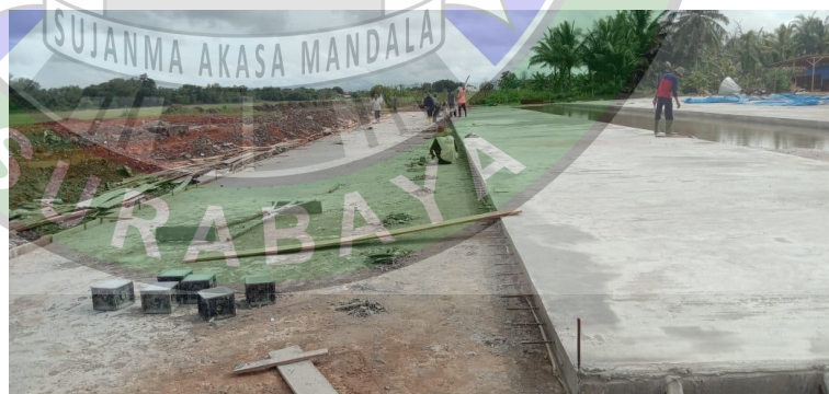
Gambar 4. 35 Proses Perawatan Beton Pasca Pengecoran
