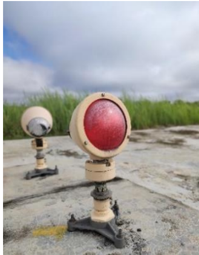
Gambar 2.18 Runway End Light Sumber: Bandara UPBU H. Asan Sampit
