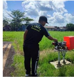
Permbersihan Lampu RTIL
