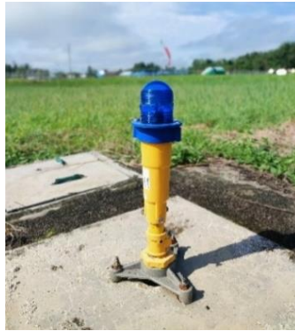
Gambar 2.22 Taxiway Edge Light Sumber: Bandara UPBU H. Asan Sampit
