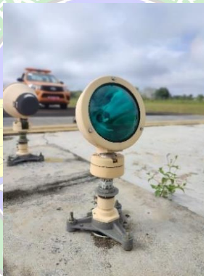
Gambar 2 19 Threshold Light Sumber: Bandara UPBU H. Asan Sampit
