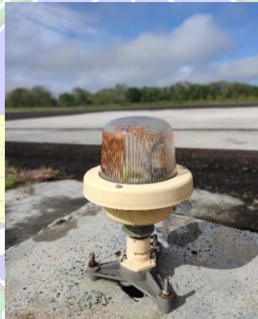
Gambar 2.20 Runway Edge Light Elevated Sumber: Bandara UPBU H. Asan Sampit
