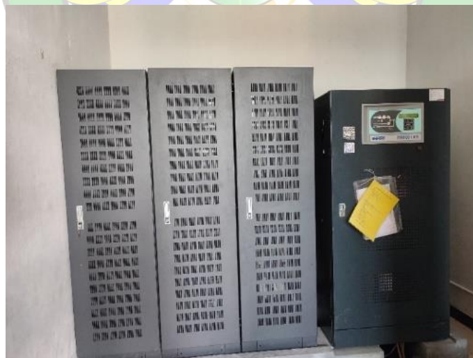
Gambar 2.7 Uninterruptable Power Supply Sumber: Bandara UPBU H. Asan Sampit
