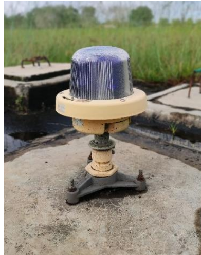
Gambar 2.23 Turning Area Light Sumber: Bandara UPBU H. Asan Sampit
