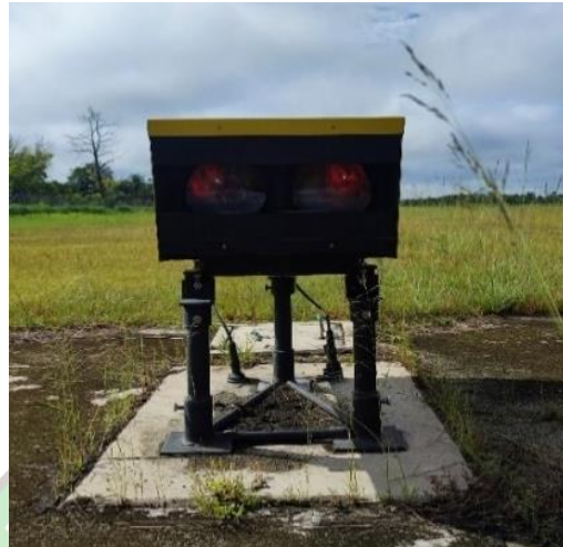
Gambar 2.15 PAPI (Precision Approach Path Indicator) Sumber: Bandara UPBU H. Asan Sampit
