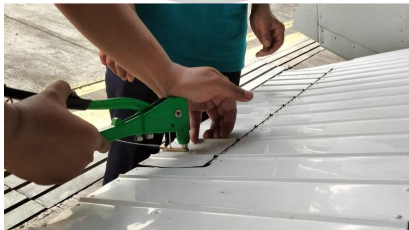
Gambar 4. 3 installation static discharge
