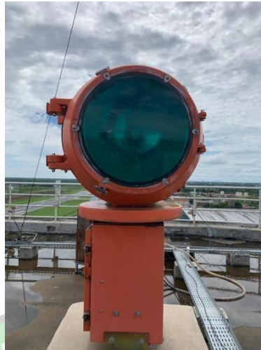
Gambar 2. 13 Rotating Beacon Light Sumber : Bandara Supadio Pontianak
