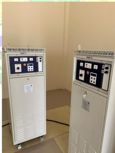
Gambar 2. 15 Constant Current Regulator
