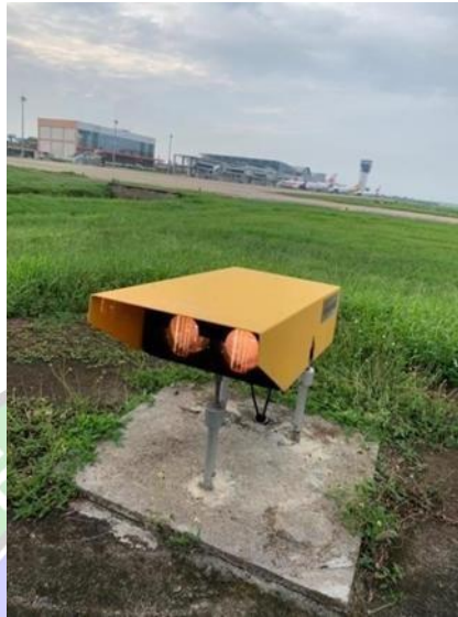
Gambar 2. 2 Precision Approach Path Indicator
