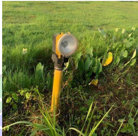
Gambar 2. 12 Sequence Flashing Light Sumber : Bandara Supadio Pontianak
