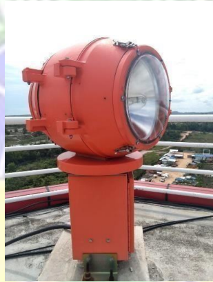
Gambar 2.27 Rotating Beacon
