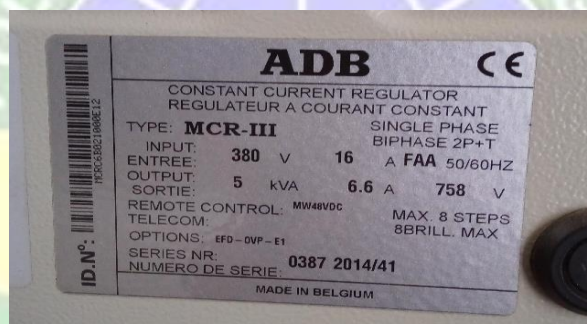
Gambar 2.36CCR Taxiway Edge Light Rangkaian C
