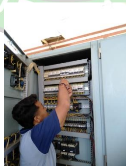
Gambar 4. 16 Re Instalasi beban
