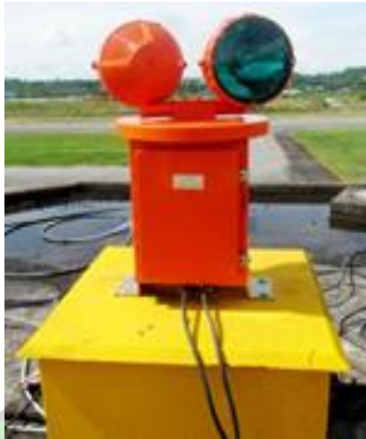
Gambar 2. 22 Rotating Beacon Sumber : Bandara Juwata Tarakan
