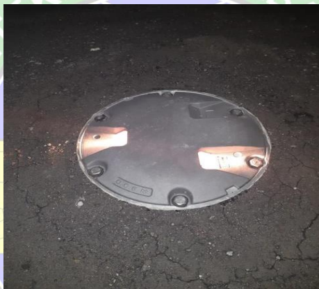
Gambar 2. 5 Runway Edge Light Insert
