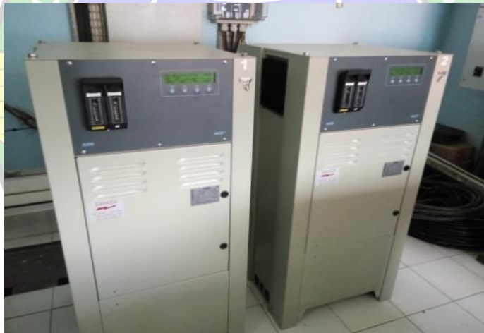
Gambar 2. 13 Constant Current Regulator (CCR) Sumber : Bandara Internasional Husein Sastranegara
