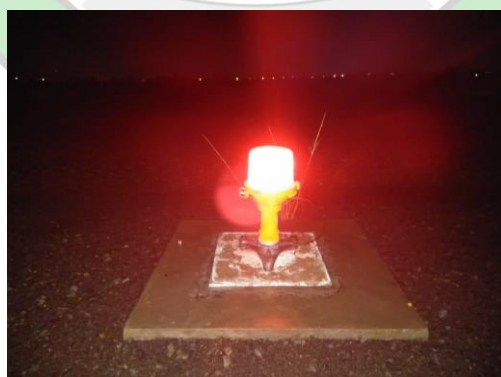
Gambar 2. 9 Runway End Light Elevated Sumber : Bandara Internasional Husein Sastranegara
