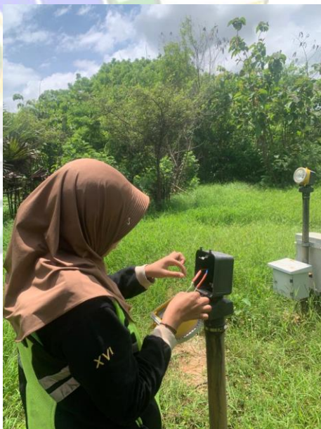
PENGgantian BOHLAM APPROACH LIGHT
