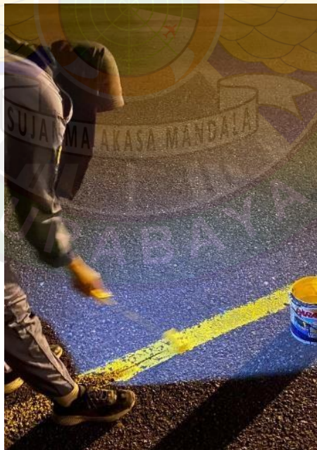
Gambar 4. 19 Pengecatan pilot stop line
