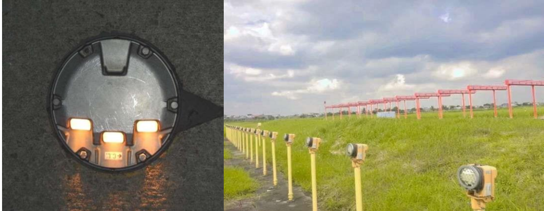
Gambar 2. 6 Approach Lighting System
