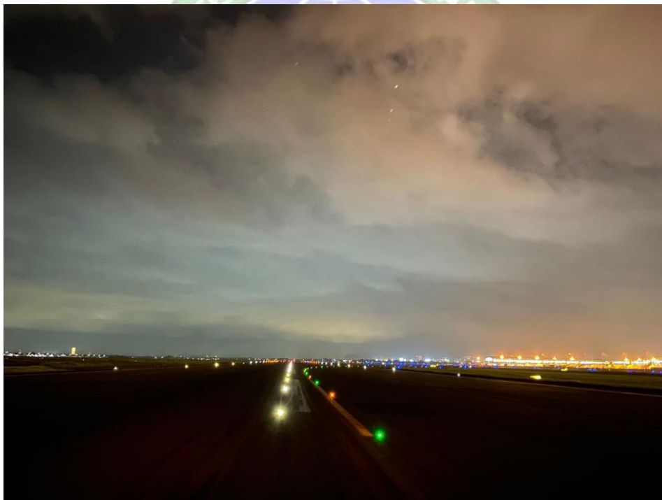
Gambar 2. 12 Exit Taxiway Centerline Light Sumber: Penulis
