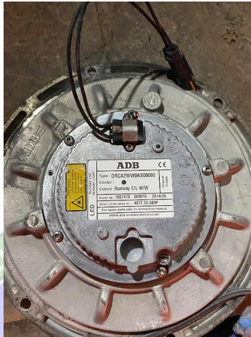
Gambar 3. 6 Armature set Runway Center Line Light inset ADB LED DRC 8 inc
