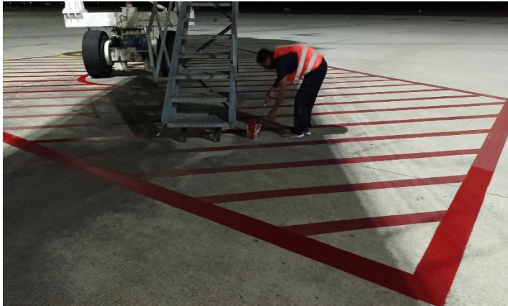
Gambar 4. 22 Pengecatan Marka Aerobridge Safety
