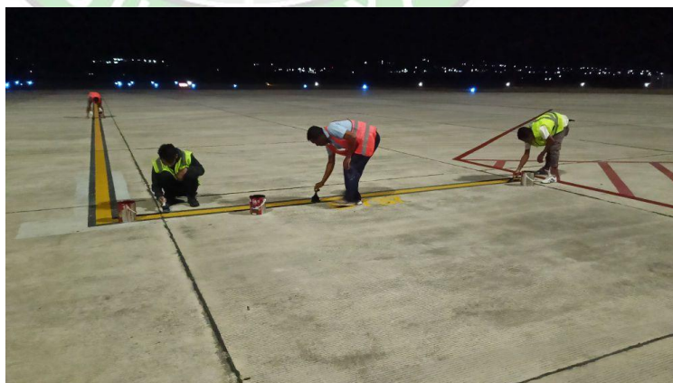
Gambar 4. 24 Pengecatan Marka Pilot Stop Line
