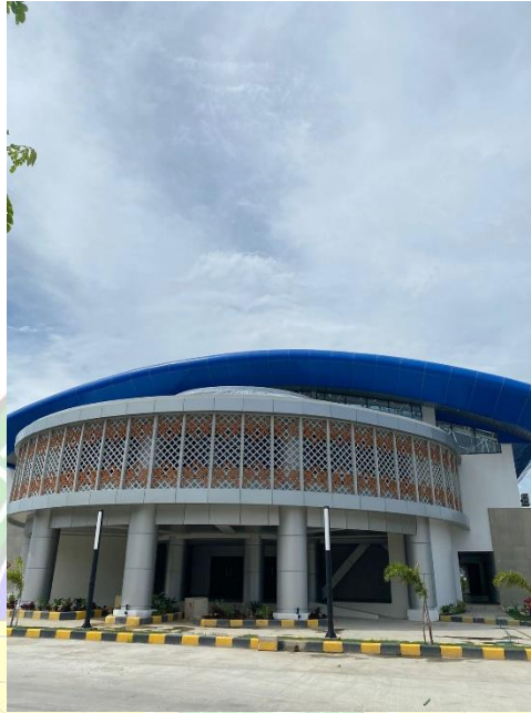
Gambar 3 10 Gedung Serba Guna (GSG)
