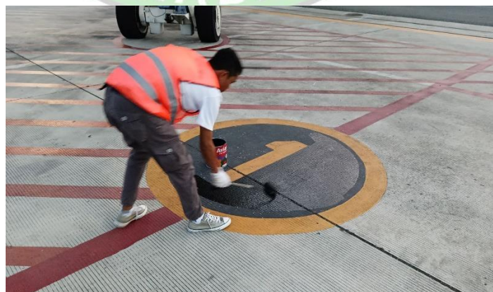
Gambar 4. 18 Pengecatan Aircraft Stand Huruf
