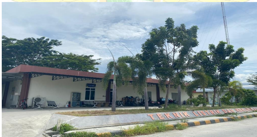
Gambar 4. 9 Gedung Power House (PH)
