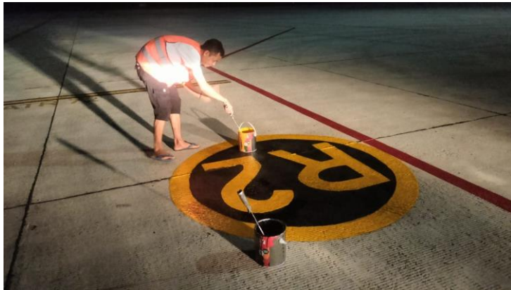
Gambar 4. 19 Pengecatan Aircraft Stand Angka
