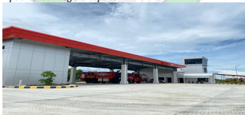
Gambar 4. 11 Gedung PKP-PK (Fire House)
