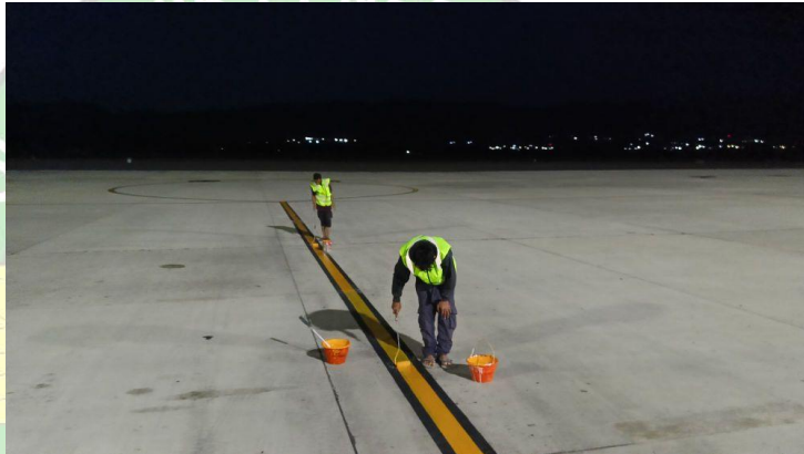
Gambar 4. 20 Pengecatan Marka Parking Stand
