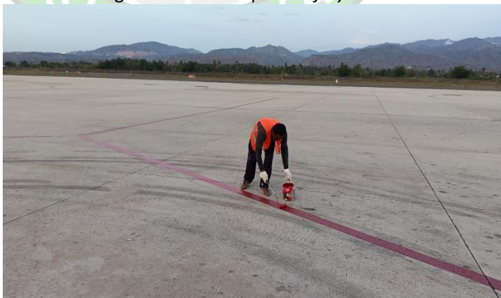
Gambar 4. 21 Pengecatan Marka Apron Safety Line
