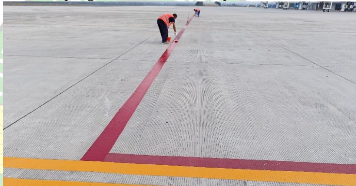
Gambar 4. 23 Pengecatan Marka Security Line
