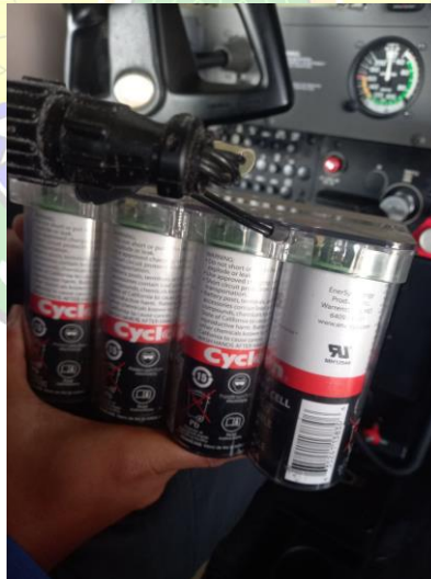
Gambar 4. 3 Inspection Standby Battery
