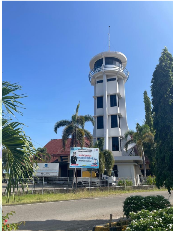
Gambar 2. 10 Menara Air Traffic Controller (ATC)
