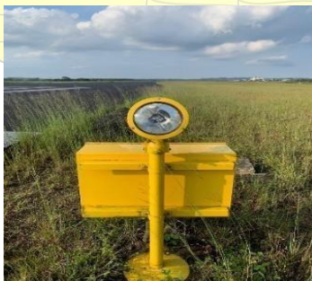
RTIL (Runway Threshold Identification Light)
