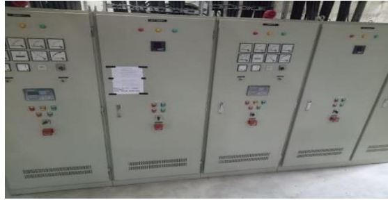
Gambar 2. 12 Panel Outgoing Sumber : UPBU A.P.T. Pranoto Samarinda
