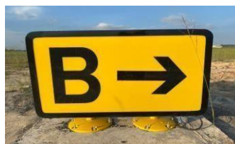
Gambar 2. 27 Taxiway Guidance Sign (TGS) Sumber : UPBU A.P.T. Pranoto Samarinda
