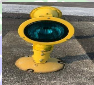
Gambar 2. 24 Elevated Threshold Light Sumber : UPBU A.P.T. Pranoto Samarinda
