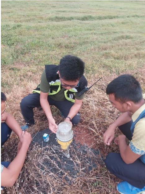
Pergantian Lampu Runway Edge Light
