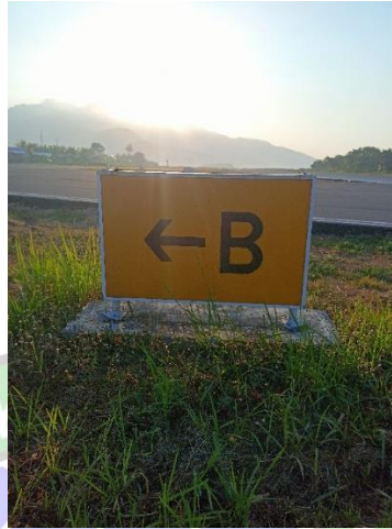
Gambar 2. 10 Taxiway Guidance Sign
