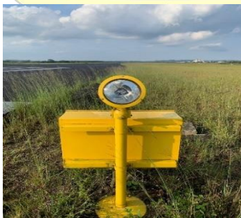
RTIL (Runway Threshold Identification Light)
