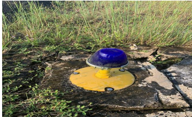
Gambar 2. 22 Turning Area Light
