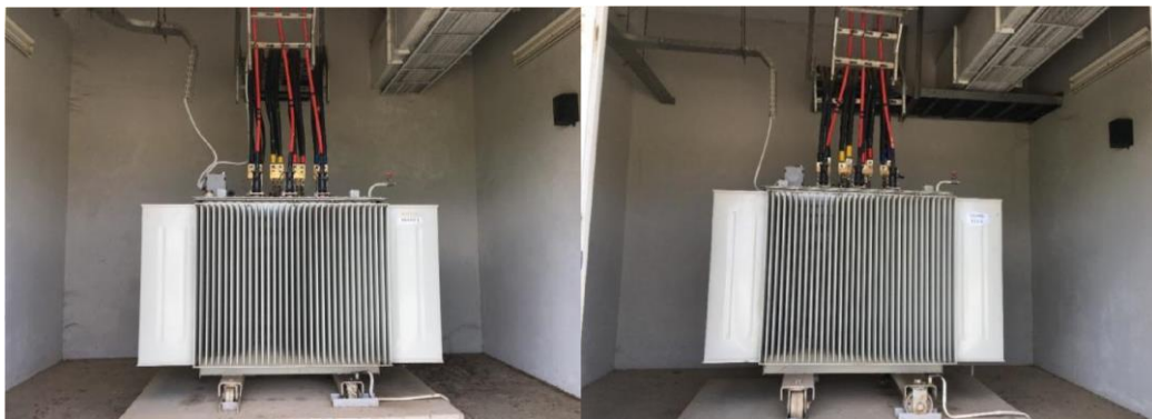
Gambar 2. 4 Tranfo Step Up& Tranfo Step Down
