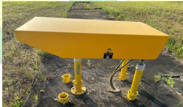
Gambar 2. 20 PAPI (Precision Approach Path Indicator)
