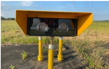
PAPI (Precision Approach Path Indicator)
