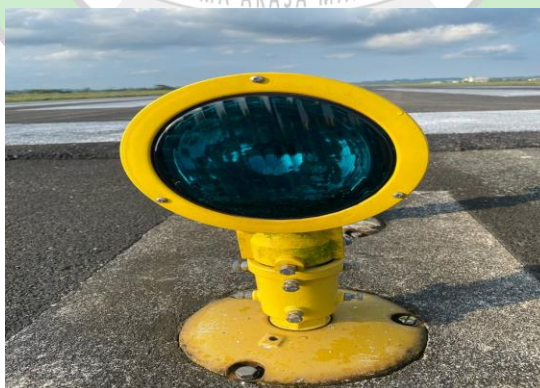
Gambar 2. 23 Elevated Threshold Light
