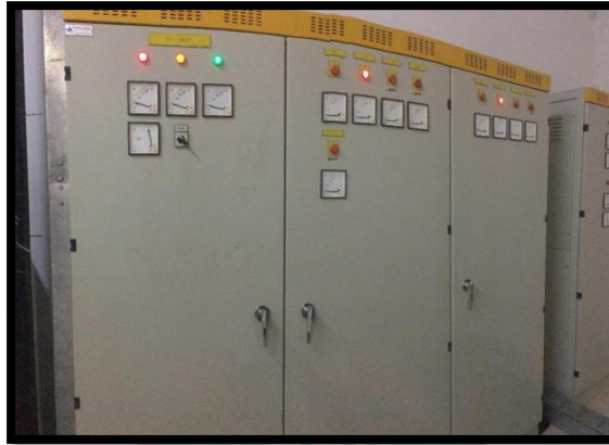
Gambar 2. 9 Panel LVMDP (Low Voltage Sub Distribution Panel)
