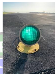
Gambar 3. 7 Lampu threshold elevated bidirectional
