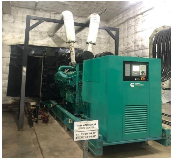
Gambar 2. 14 Power Generation Cummins
