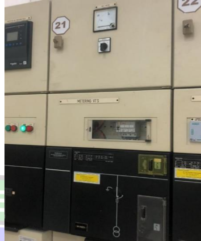
Gambar 2. 18 Panel Metering
