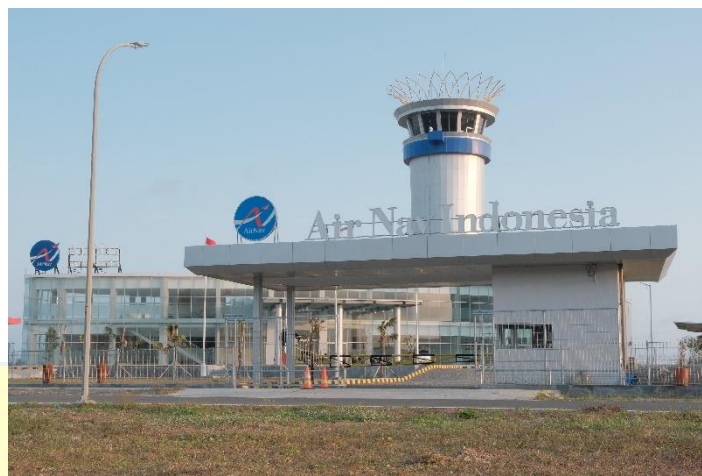
Gambar 2. 9 Menara Air Traffic Controller (ATC)
