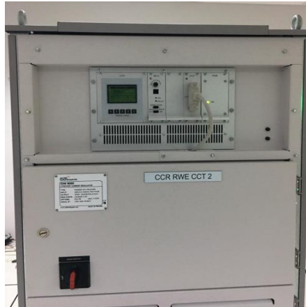
Gambar 2. 27 Constant Current Regulator
