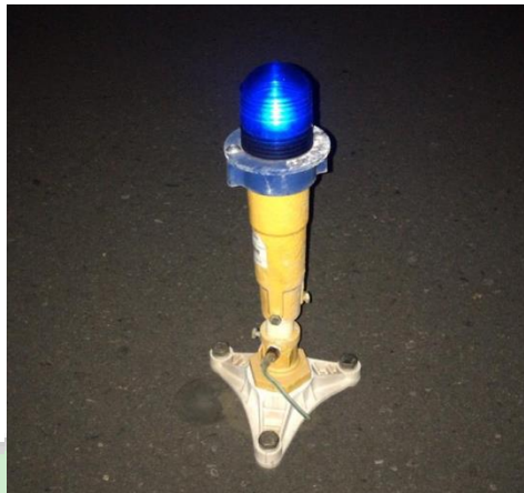
Gambar 2. 18 Taxiway Edge Light
