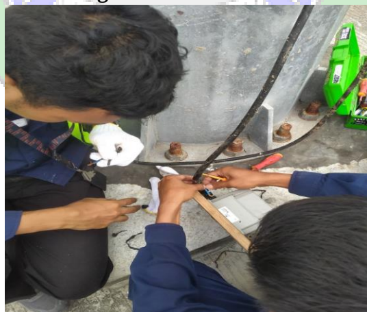
Penggantian Lampu Flood Light
