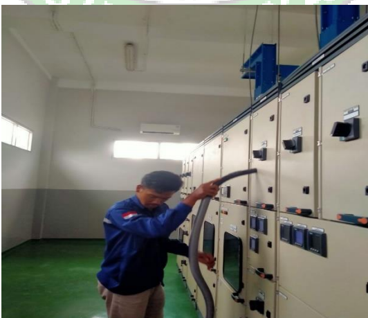
Pembersihan Panel Sub Station
