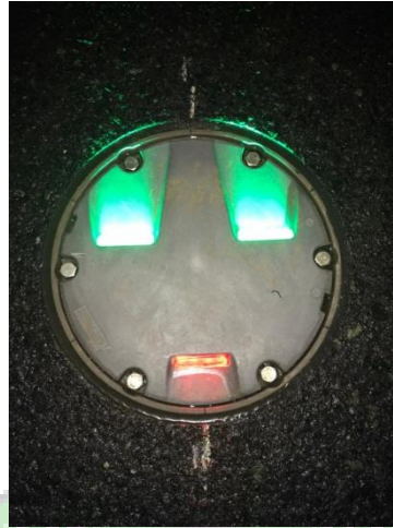
Gambar 2. 16 Runway Threshold Light
