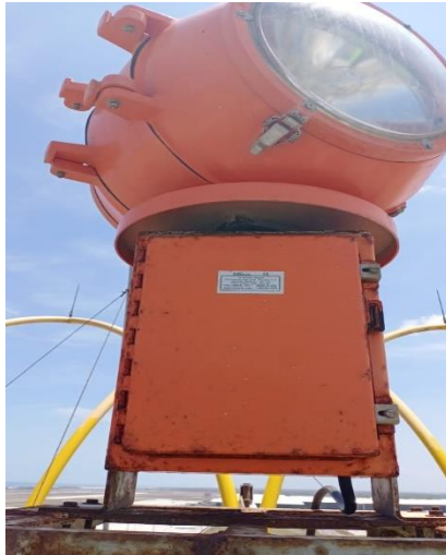
Gambar 2. 24 Rotating Beacon
