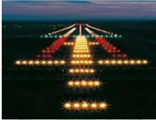
Gambar 3. 1 Lampu Airfield Lightning System
