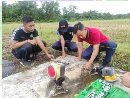
Penaikan Lampu Threshold
