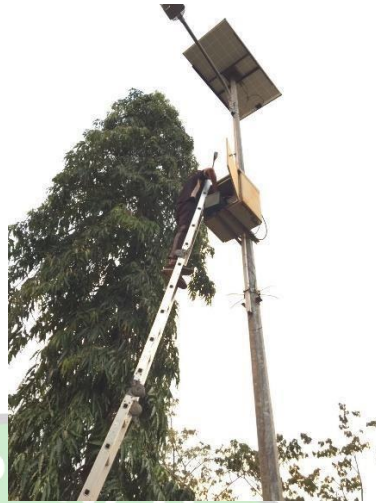
Pergantian Battery Lampu Jalan
