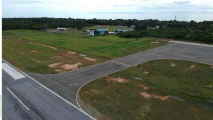
Gambar 2. 4 Taxiway UPBU Sangia Nibandera Kolaka
