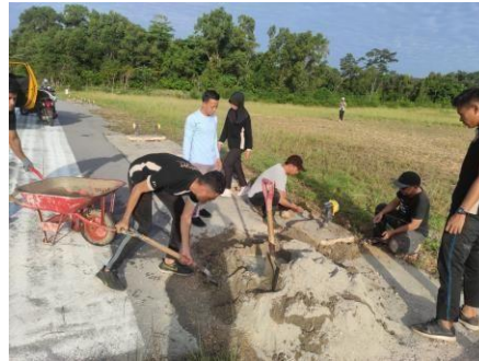
Pengecoran Lampu Treeshold
