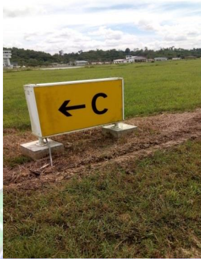
Gambar 2. 33 Taxiway Guidance Sign
