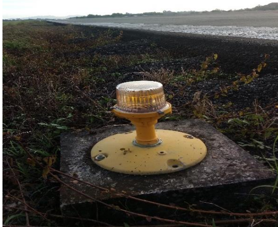
Gambar 2. 23 Gambar 2.20 R/W Edge Light
