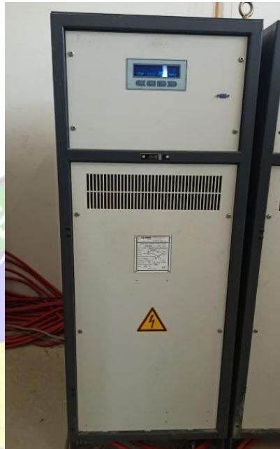
Gambar 2. 20 CCR ( Constant Current Regulator)
