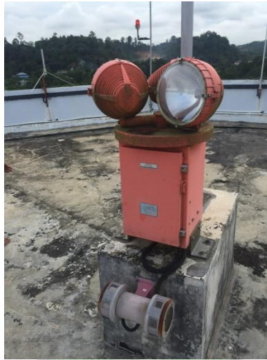
Gambar 2. 27 Rotating Beacon
