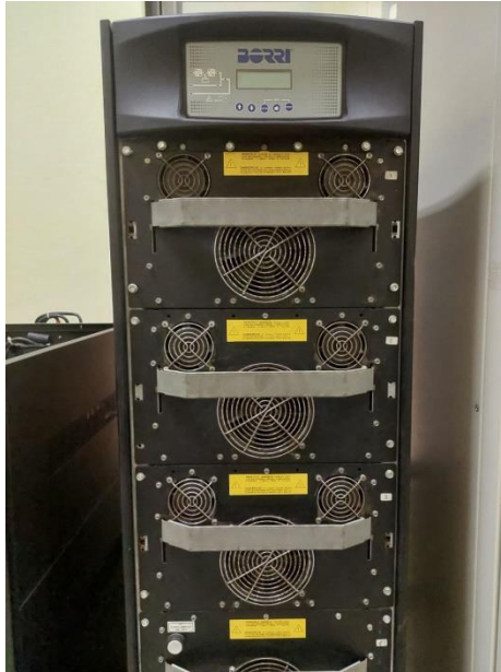
Gambar 3.1 UPS BORRI B8033FXS Sumber: Bandara H. Hasan Aroeboesman
