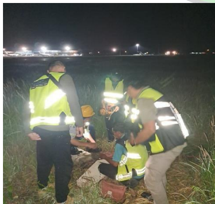
Gambar 5. 7 Cek Trafo taxiway
