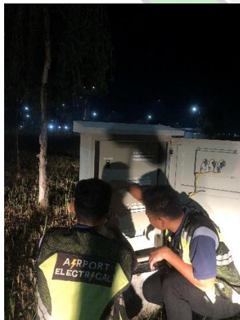
Perawatan dan Pengecekan Panel PJU
