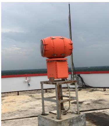
Gambar 2. 17 Rotating Beacon
