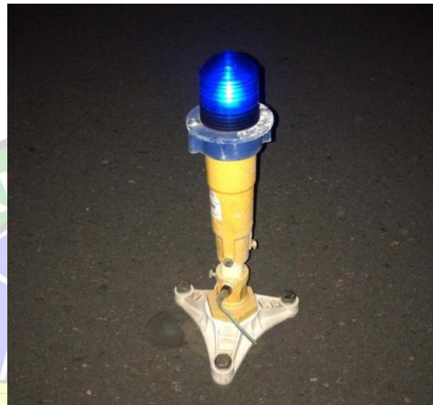
Gambar 2. 10 Taxiway Edge Lights
