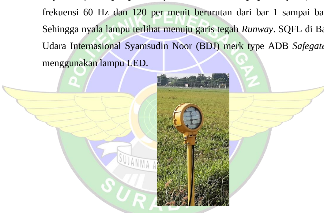
Gambar 2. 3 Sequence Flashing Light (SQFL)
