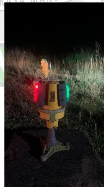
Gambar 2. 6 Threshold Light dan Runway End Light Elevated
