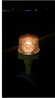
Gambar 2. 7 Runway Edge Lights
