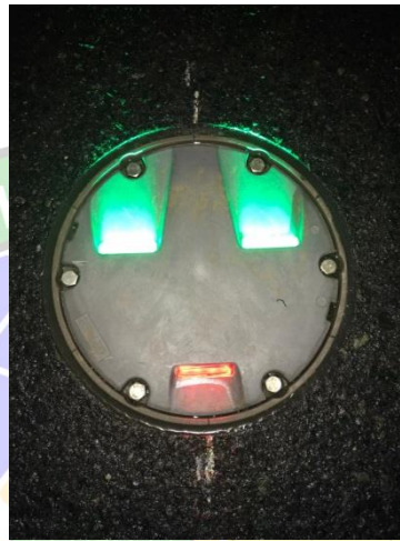
Gambar 2. 5 Threshold Light dan Runway End Light Insert
