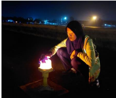
Perawatan Runway Edge Light
