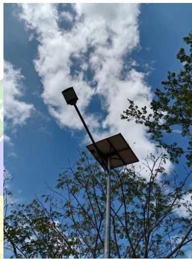
Gambar 4. 10 PJU Berbasis Solar Cell
