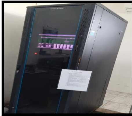
Gambar 2. 24 Marshalling Cabinet
