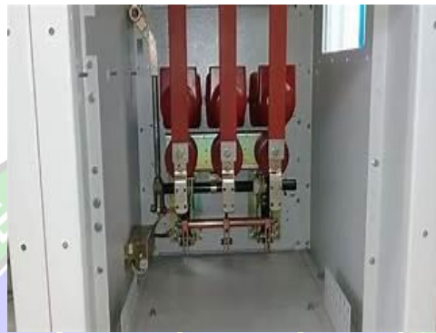
Gambar 3. 24 Earthing Switch
