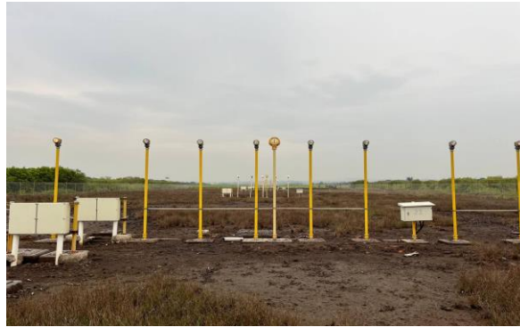
Gambar 2. 12 PALS ( Precision Approach Light System ) CAT 1
