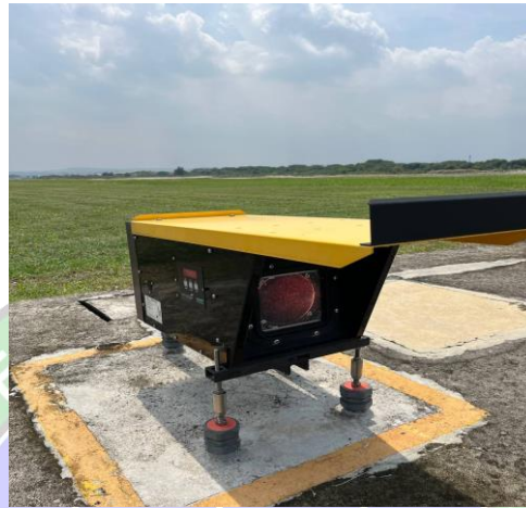
Gambar 2. 14 Precision Approach Path Indicator (PAPI)
