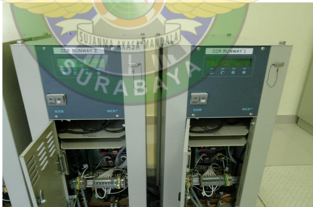
Gambar 2. 6 Constant Current Regulator (CCR) Runway Light
