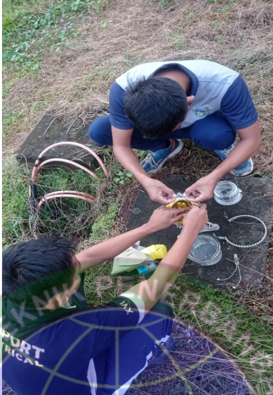
Pergantian lampu halogen Runway edge light
