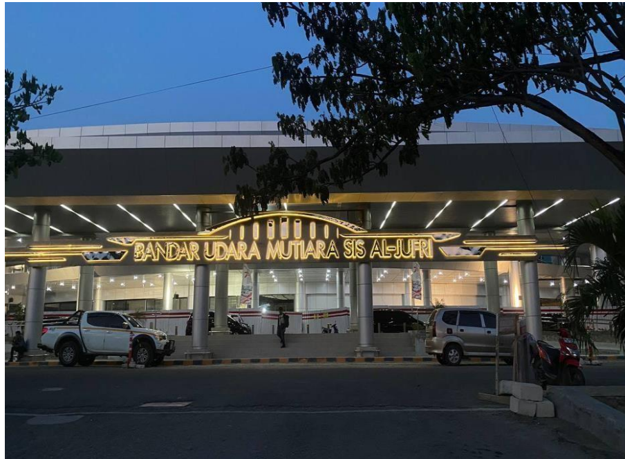
Gambar 1.1 Terminal Bandara Mutiara Sis Al-Jufri
