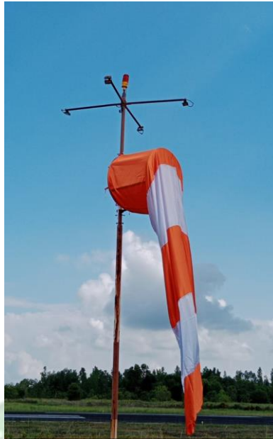
Gambar 2. 26 Wind Direction Indicator Light Sumber : Bandara Internasional Juwata Tarakan
