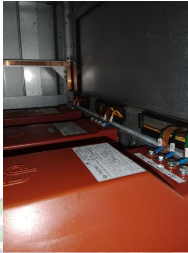
Gambar 3. 8 Current Transformer
