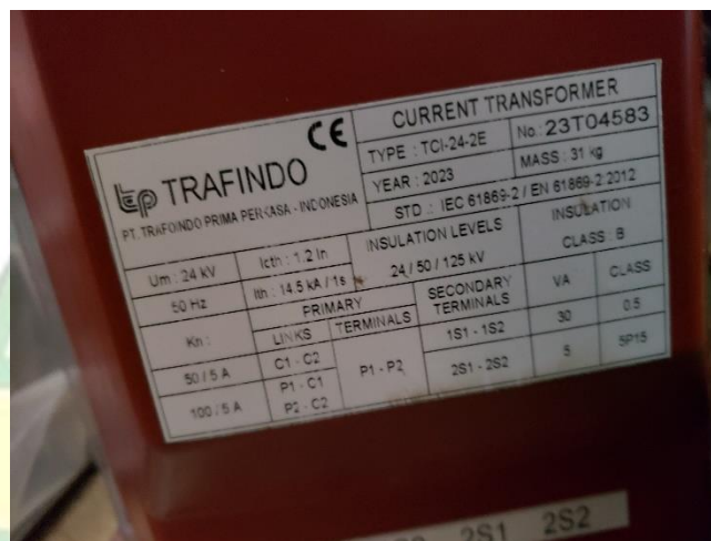
Gambar 4. 4 Gambar nameplate CT
