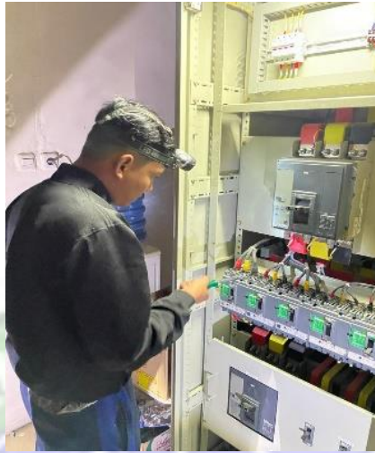
Gambar 4.1 Melepas MCCB pompa hydrant 100 A
