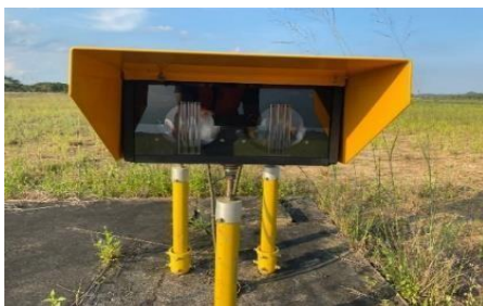
PAPI (Precision Approach Path Indicator)
