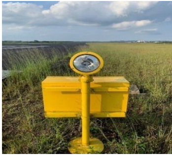
RTIL (Runway Threshold Identification Light)
