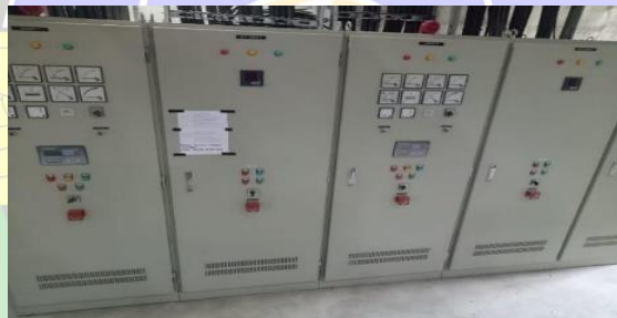
Gambar 2. 12 Panel Outgoing Sumber : UPBU A.P.T. Pranoto Samarinda
