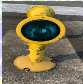
Gambar 2. 24 Elevated Threshold Light Sumber : UPBU A.P.T. Pranoto Samarinda
