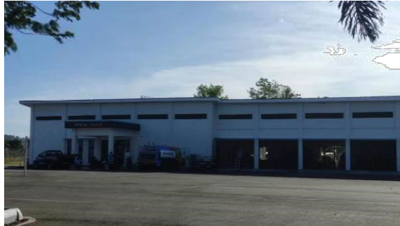
Gambar 4.12 Gedung Power House
