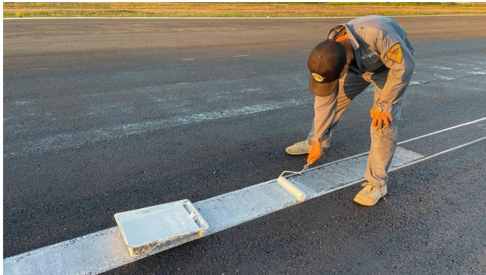
LAMPIRAN 17 : PENGECATAN MARKA RUNWAY (CENTERLINE)
